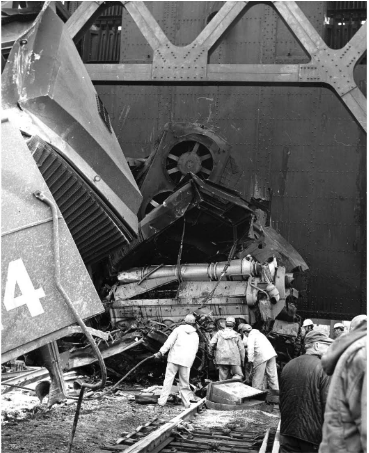
The massive counterweight can be seen behind crews working to remove locomotive components. Notice the fans on the top of the unit, top center.
